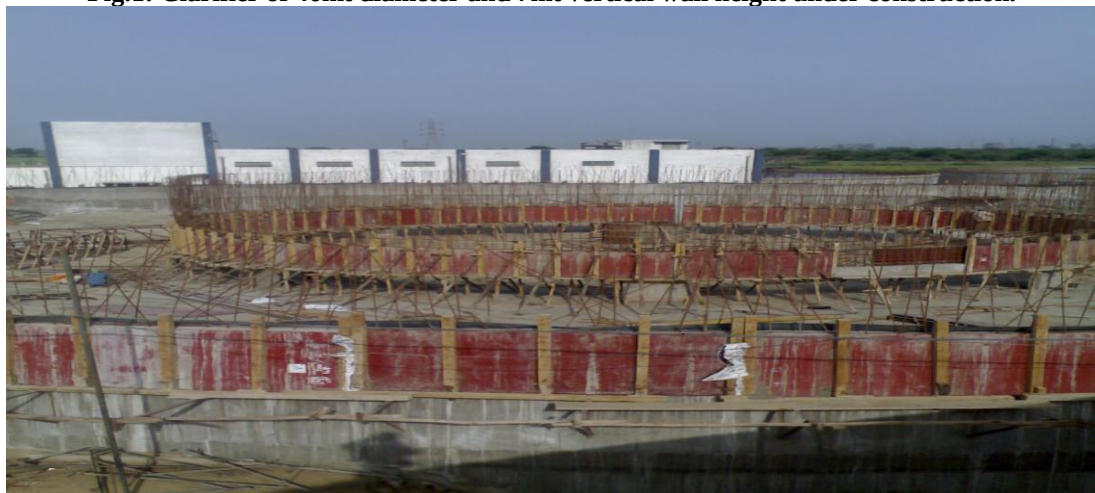
Fig.1: Clarifier of 46mt diameter and 7mt vertical wall height under construction.
