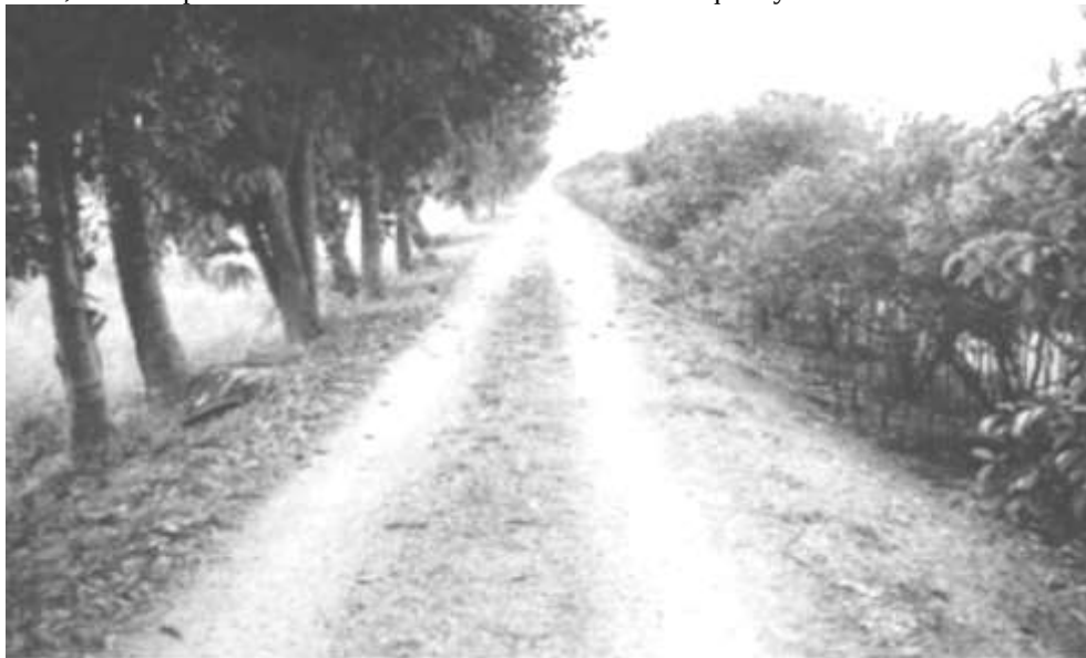
Plate I, Laterite road surface [15]
