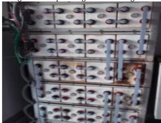
Figure 6: Battery Bank of a BTS site
