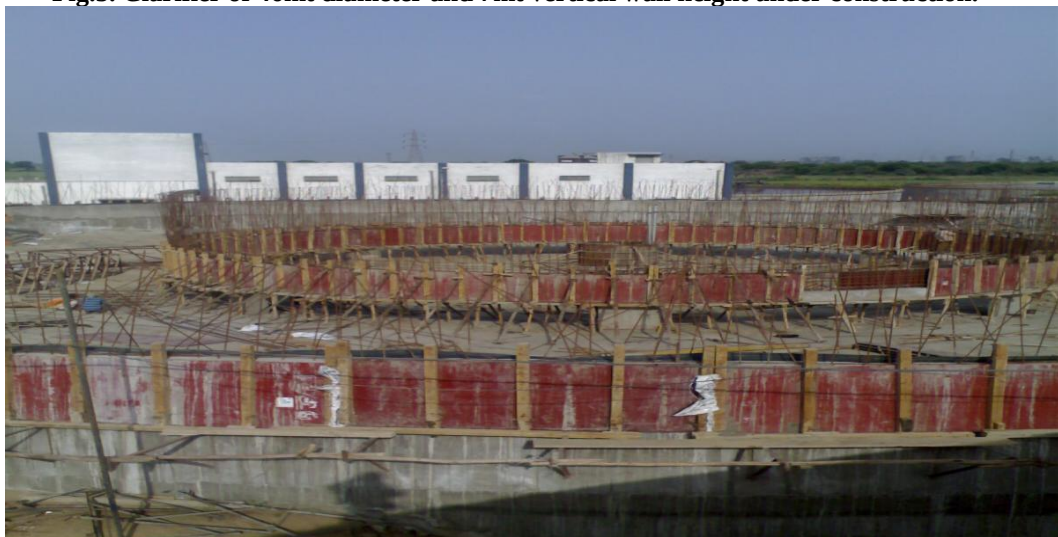
Fig.5. Clarifier of 46mt diameter and 7mt vertical wall height under construction.
