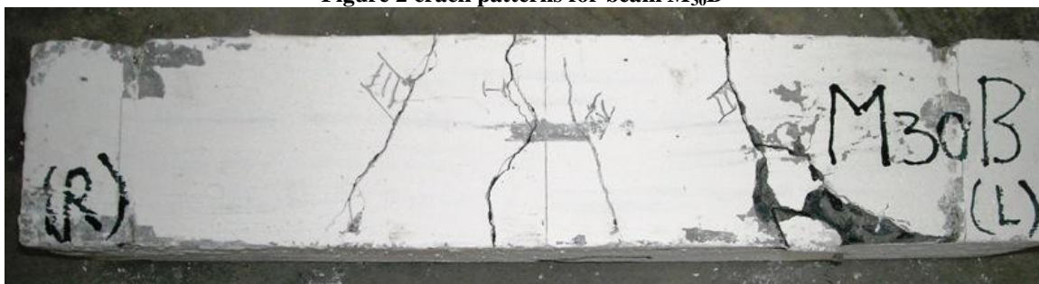
Figure 2 crack patterns for beam M_{30}B
